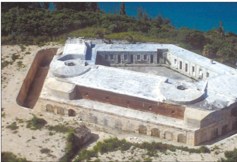
The iron-fronted Fort Cunningham, modified in the 1870s on the original 1820s base.
